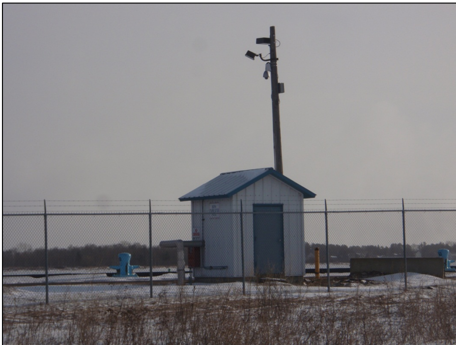
Photo 1: Building for the Bow Thruster Pump
