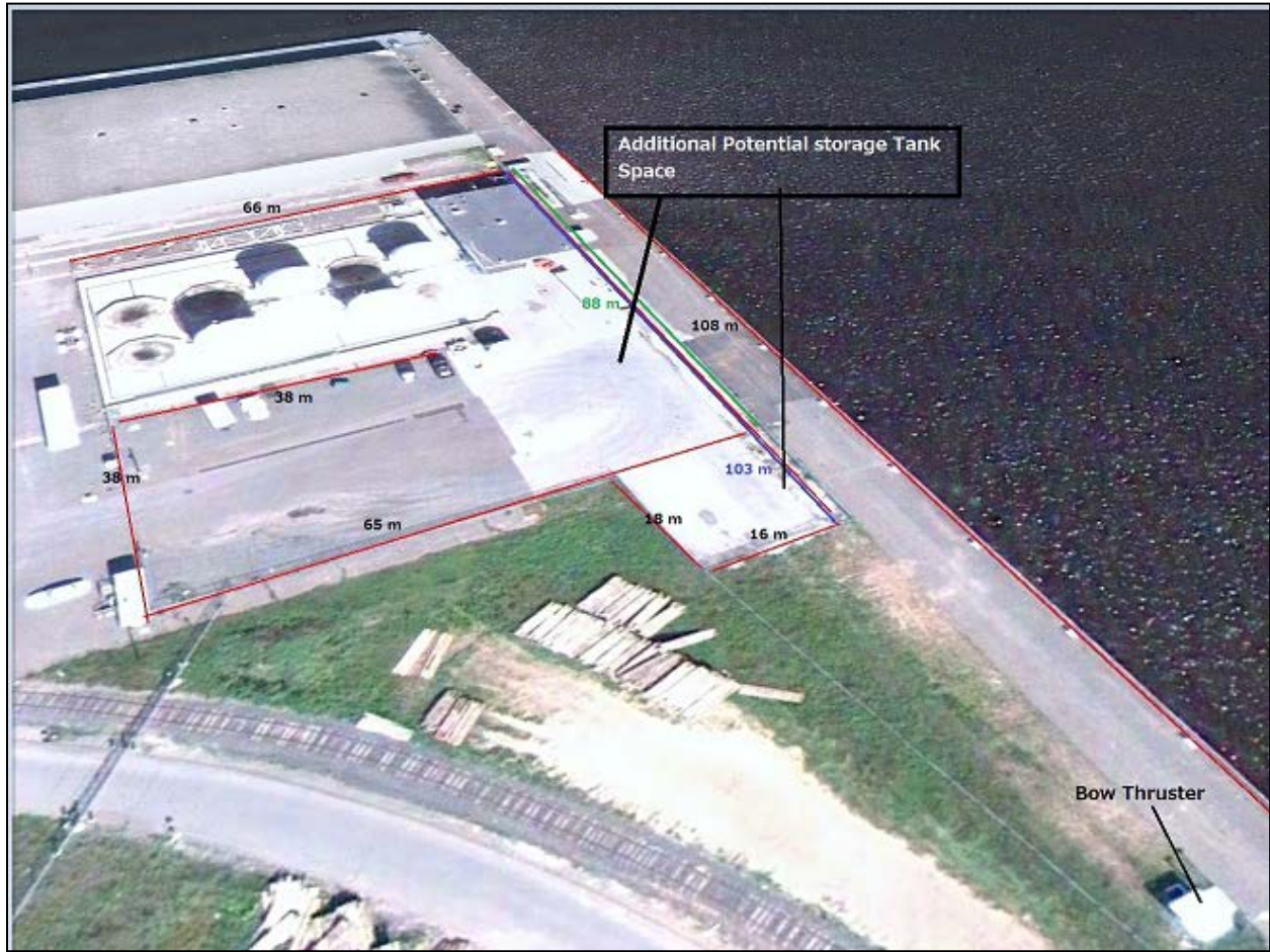
Photo 4: Additional Potential Storage Tank Location
