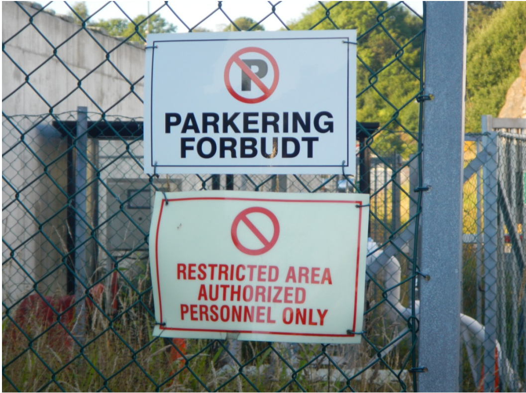
Figure 5 LNG Storage Tank Fencing and Warning Signs
